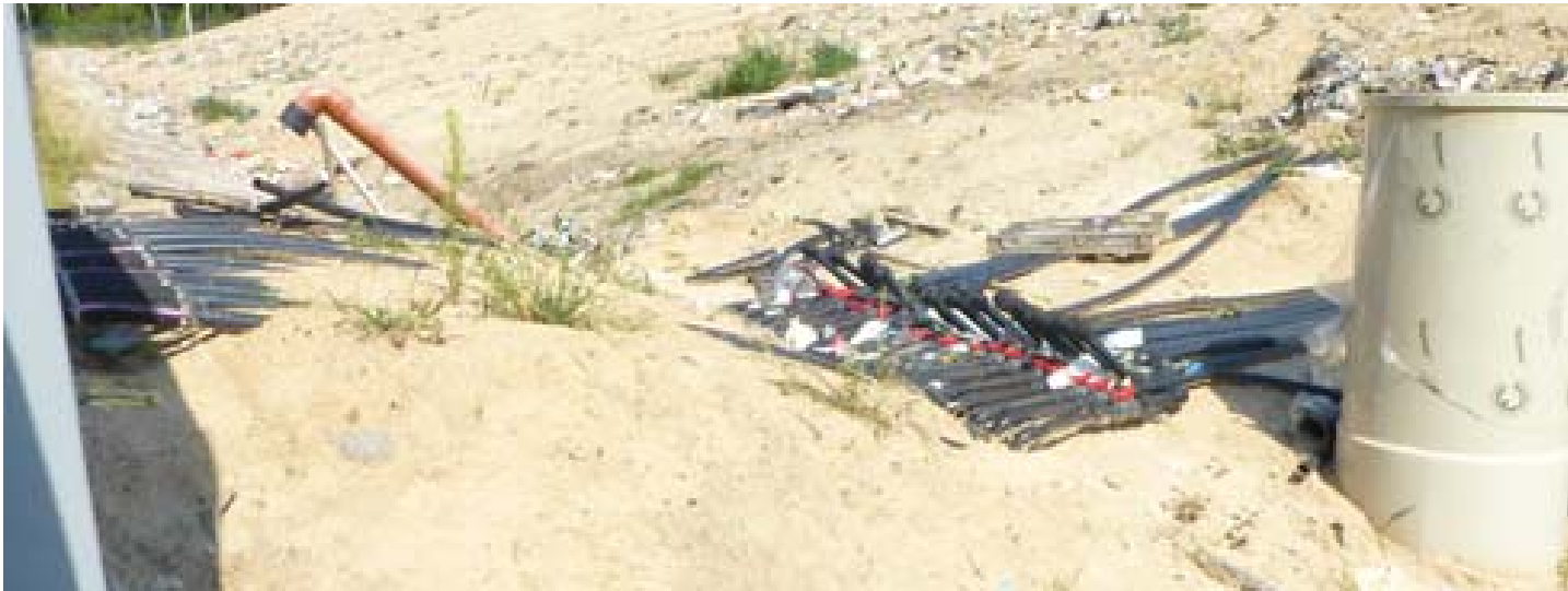
Manifold station on the brink of the landfill with dewatering (to the condensate shaft) and purge connections
